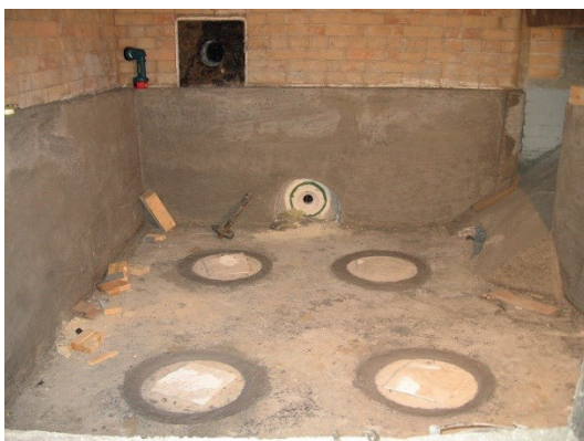
Installation of gas diffusers in an aluminium melting furnace.
